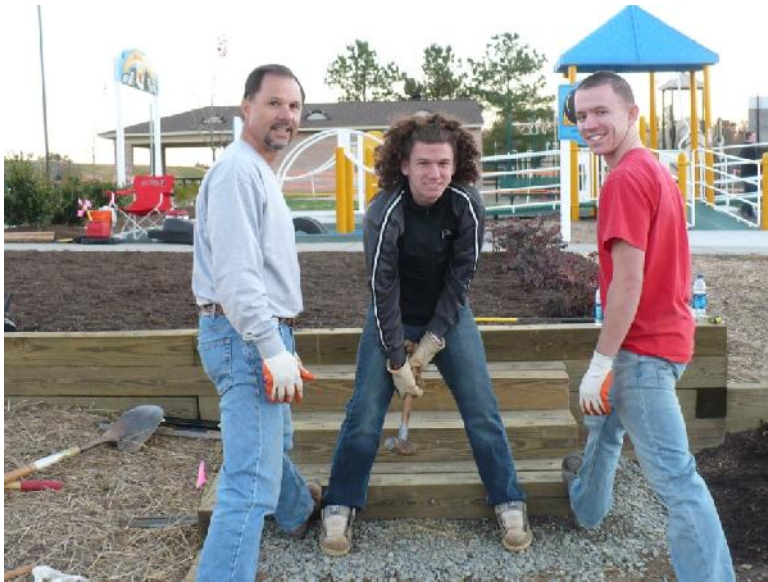
Hammering in the last rebar!
