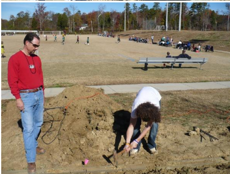
Hammering in the rebar.
