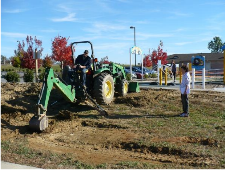
Grading the hill.
