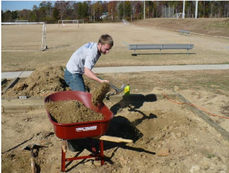
Smoothing out the first level.
