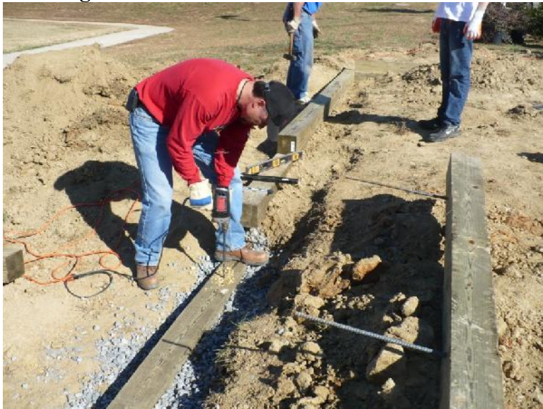
Digging the trenches for the retaining wall.
